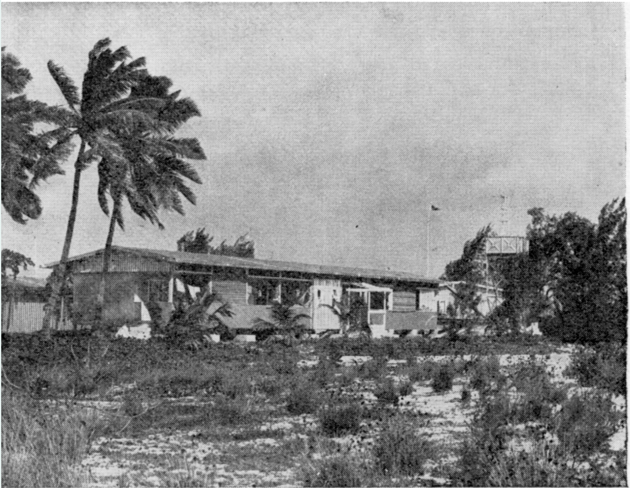
FIGURE 1. The Aldabra Research Station from the northwest.
